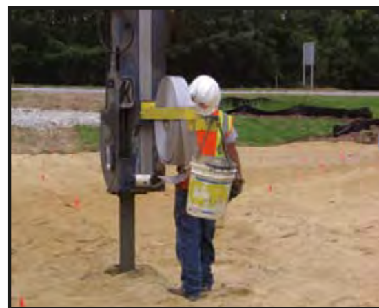
Installation of Prefab. Vertical Drains
