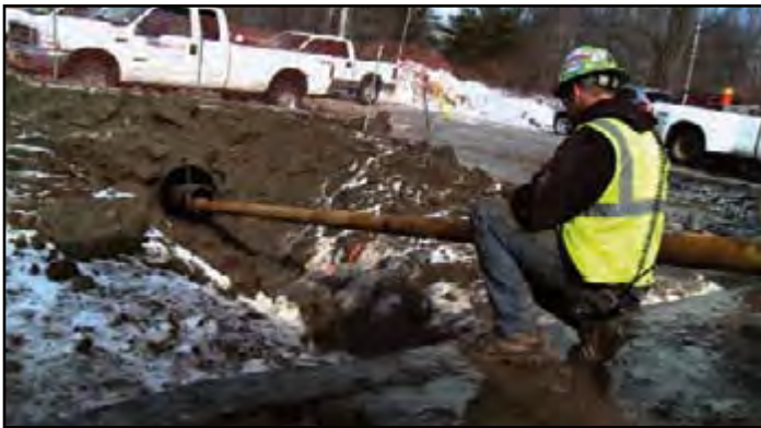
Drill Enters the Casing
