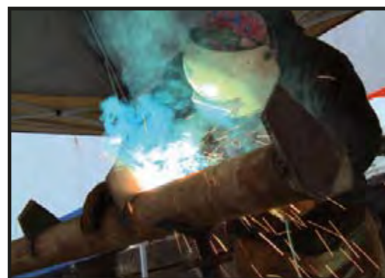
Welder Preparing for Installation of Drains
