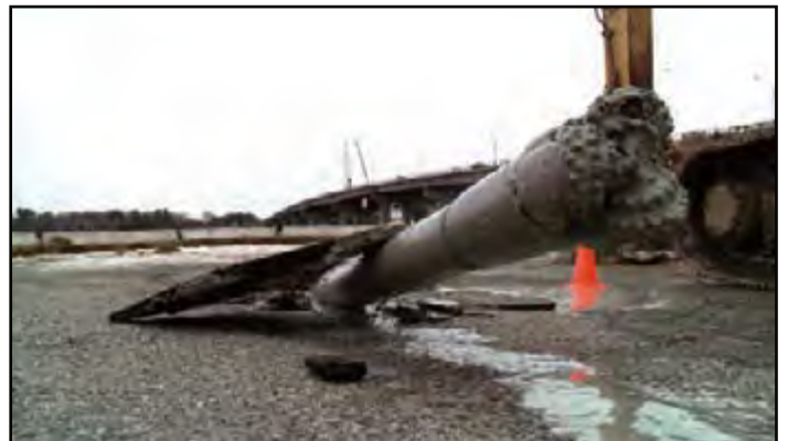
Pilot hole, Dover Point
