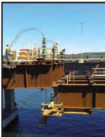
Erection of the Middle Span
