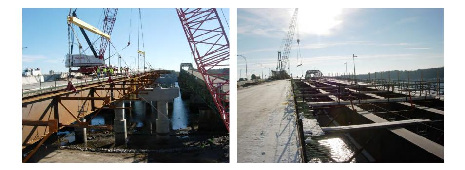
Work Underway – Phase 2 Newington Abutment The last major concrete foundation piece that needs to be completed is the Phase 2 Abutment Wall on the Newington side of the bridge. This work is currently underway.
