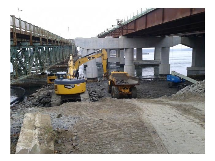
Work Underway – Phase 2 Structural Steel Erection Work began in December of 2012 constructing the westerly half of the bridge including 3 additional steel girders which will be erected from the Phase 1 bridge deck. This work will continue into March of 2013.
