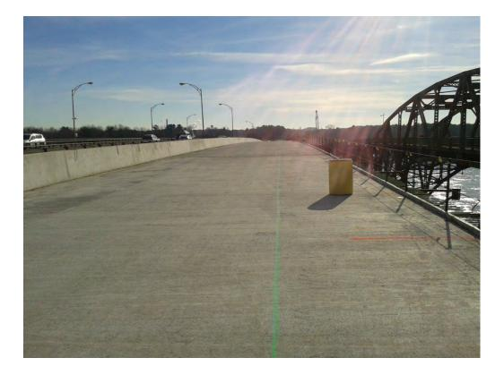
Work Completed – Phase 2 Pier Concrete Work Phase 2 constructs the westerly half of the bridge including the construction of one additional support column and an additional section of the pier cap. Phase 2 Pier concrete work was completed in the fall of 2012 and is ready to receive the structural steel girders.
