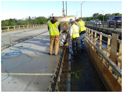
Epoxy coated steel reinforcement has been installed over the entire bridge deck in preparation for the 5" concrete overlay which will be completed by the end of June.
