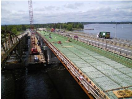
Work on Phase 1 is almost complete. Cianbro Corporation will start Phase 2 work in July of 2012. Phase 2 will build the west half of the bridge and includes additional pier construction work.
