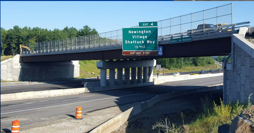
Woodbury Avenue Bridge – looking NB
