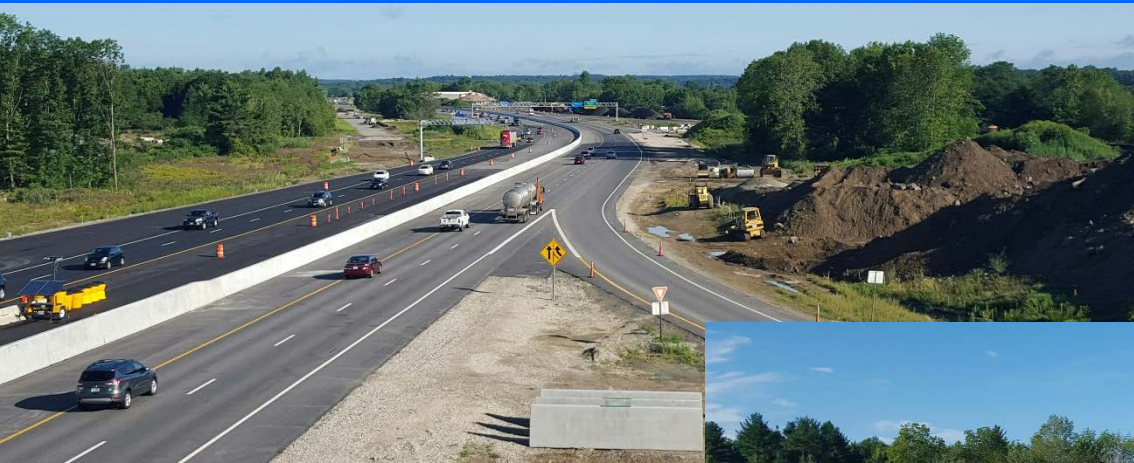
Exit 3 NB On Ramp
