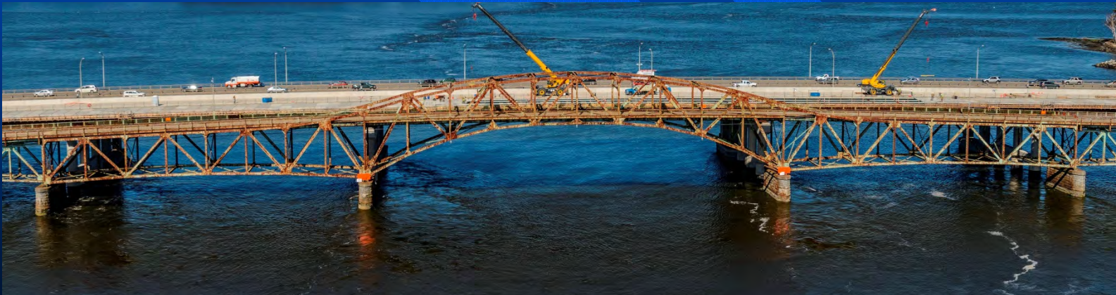
Spans 4-5-6 (Center Spans)
