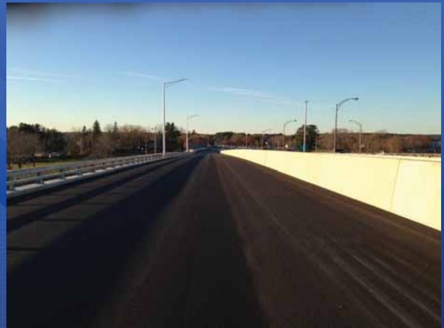
Final Bridge Deck (2013)
