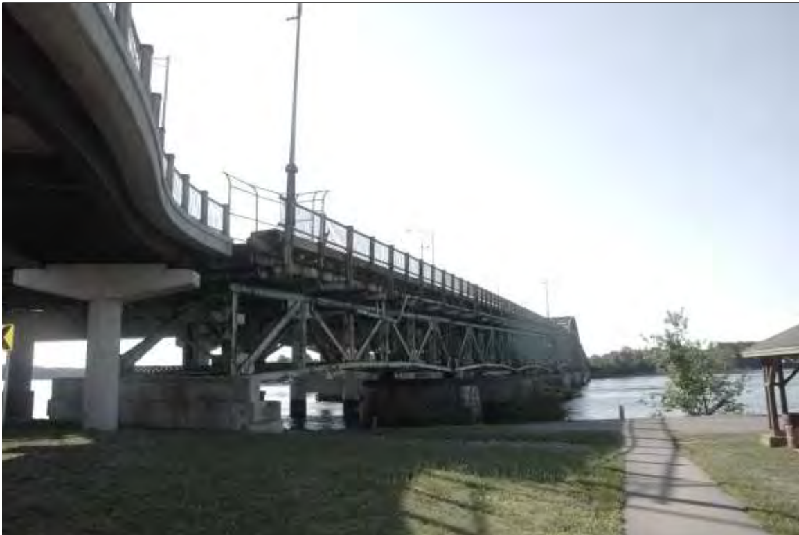
Photo # 3 Description: General Sullivan Bridge with new north approach (left) and picnic pavilion (right) Reference (file name or frame#): DOV0150_3
