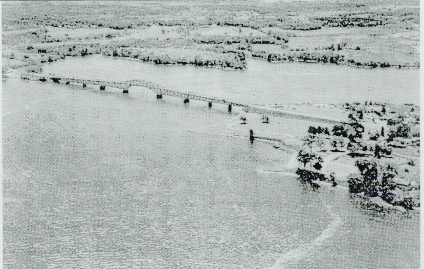
General Sullivan Bridge Before Construction of Little Bay Bridge, Hilton Park at right (Bunker 2002)
