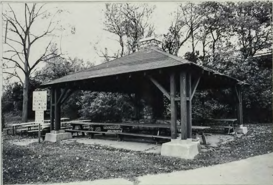
Photo 2: Picnic pavilion and Sullivan Bridge abutment (southern section of park)
