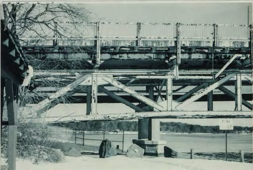
Photo 4: Sullivan Bridge and connecting walkway (southern section of park) Roll: 2005-7 Frame: 9 Direction: E
