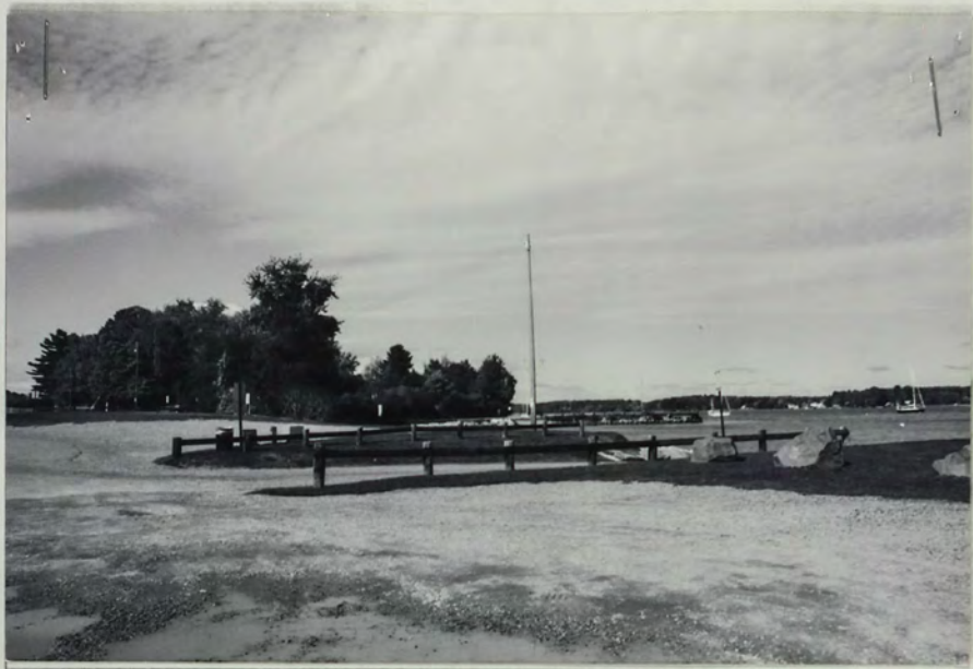
Photo 14: Boat ramp and Piscataqua River
