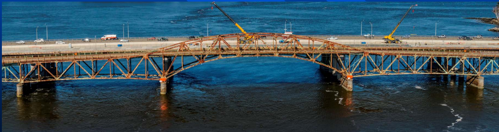
Spans 4-5-6 (Center Spans)
